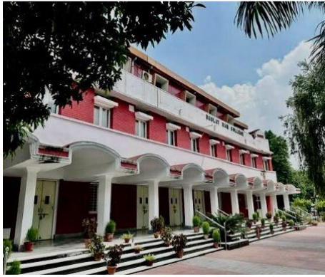
Well ventilated building structure
